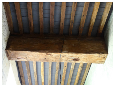
RDC – couloir Buffon
